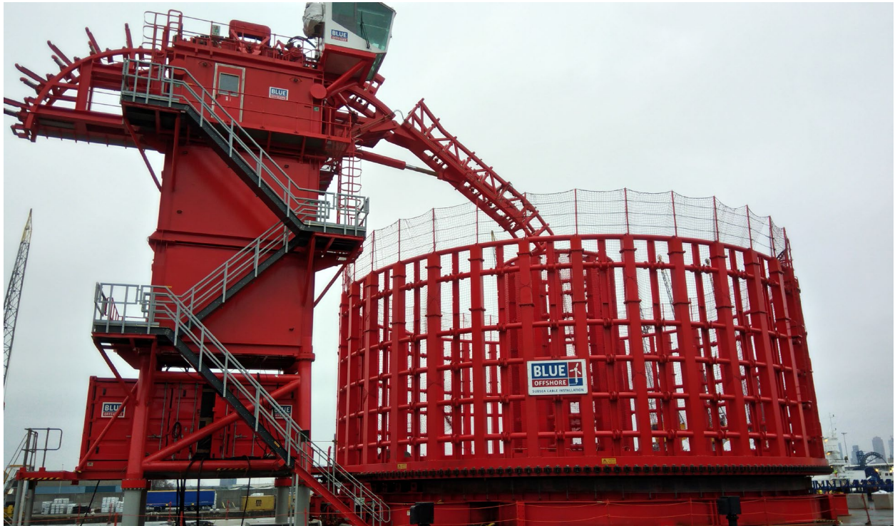
Figure 2 • Blue Offshore's BC01 23m OD, basket carousel 10m fill height and loading tower 18m total height.
