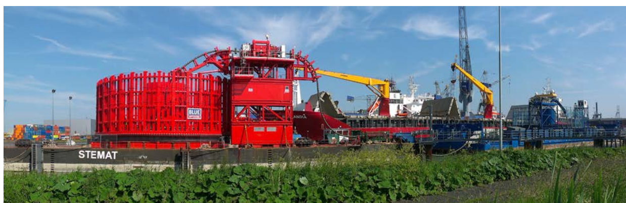
Figure 1 • Cable loading of Blue Offshore's system 'BC02' on storage barge Stemat 92.
