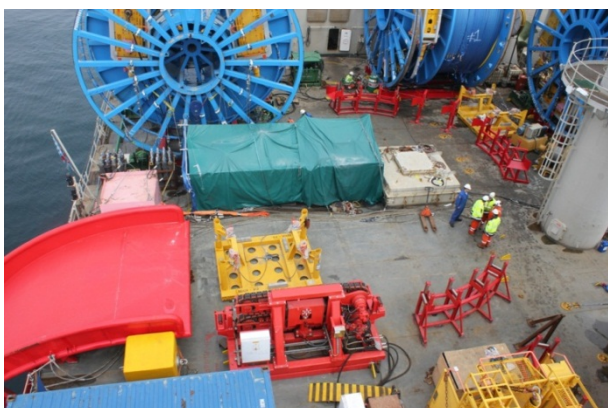
Figure 5 • Ready for umbilical installation.
